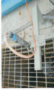
Sampling pump at Effluent
